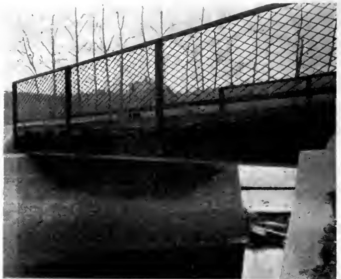
A standard type of steel I-beam bridge.—A 30-ft. span in the Municipality of Lorne
